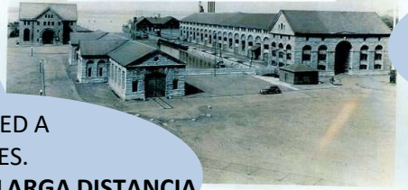
Niagara Falls power Co. 1895 The first major hydro-electric power plant in the world Adams Station, power houses #1+ #2 and transformer building
